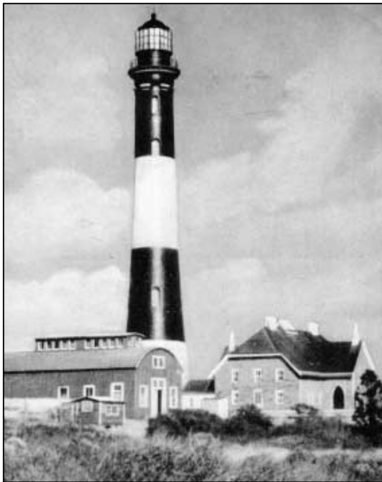
Fire Island Lighthouse
