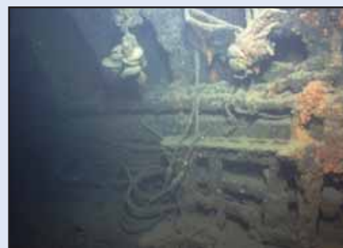
The port side of the control room
