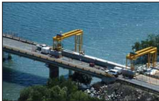
Elizabeth River Rail Bridge
