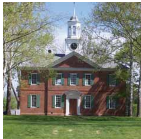
The Chowan County Courthouse
