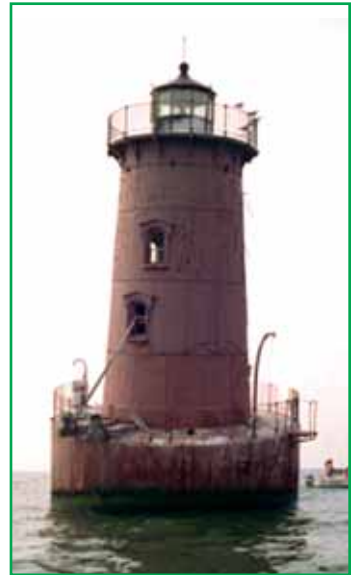
Sharp's Island Lighthouse
