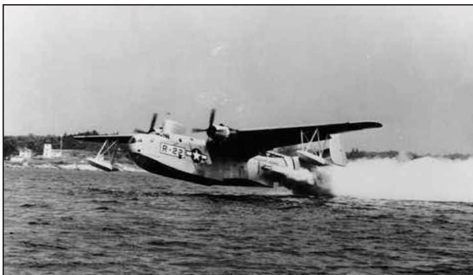
A U.S.C.G. Martin Mariner rocketing from the water with JATO.
