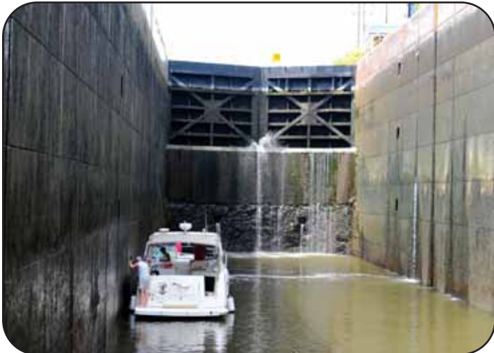
Erie Canal Mohawk River lock with 35’ lift.
