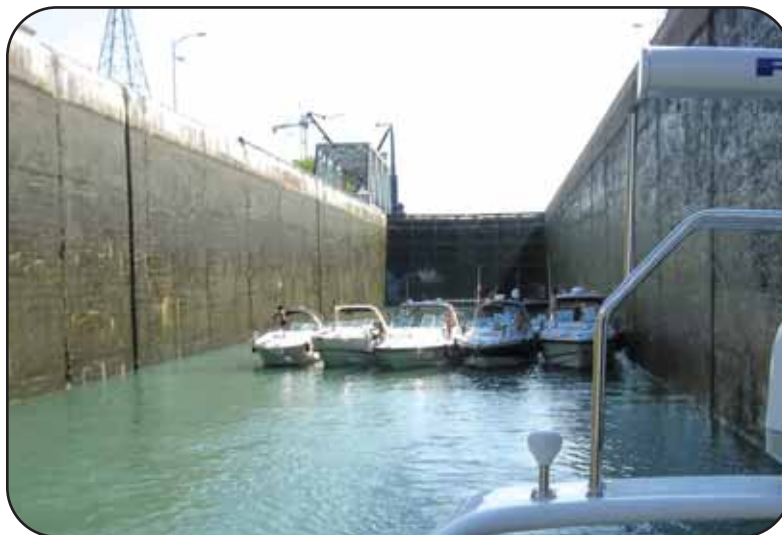
St. Lawrence Seaway commercial locks where pleasure boats must raft when locking.
